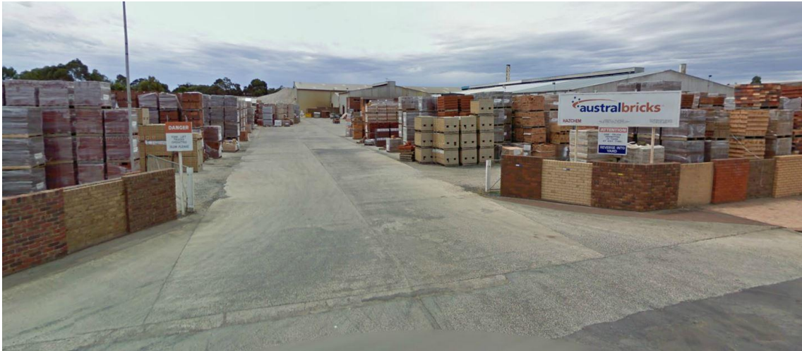
Figure 2: View of Longford plant storage yard (Source: Google maps)
